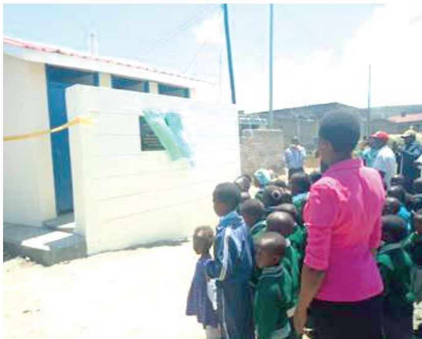
The pit latrines constructed usin fairtrade premiums by bigot farm
