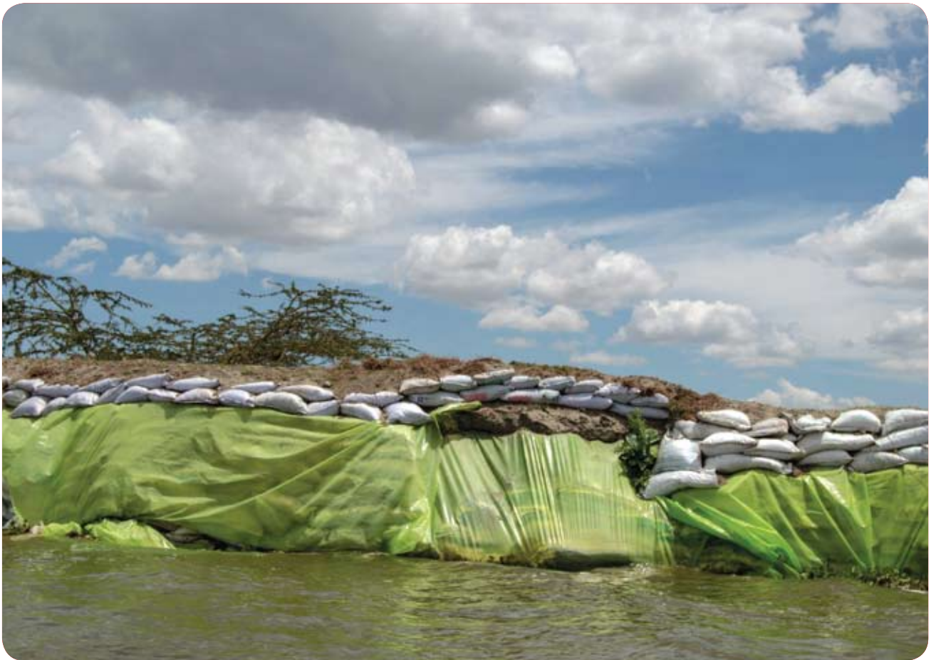
A dike constructed within the lake by an investor
