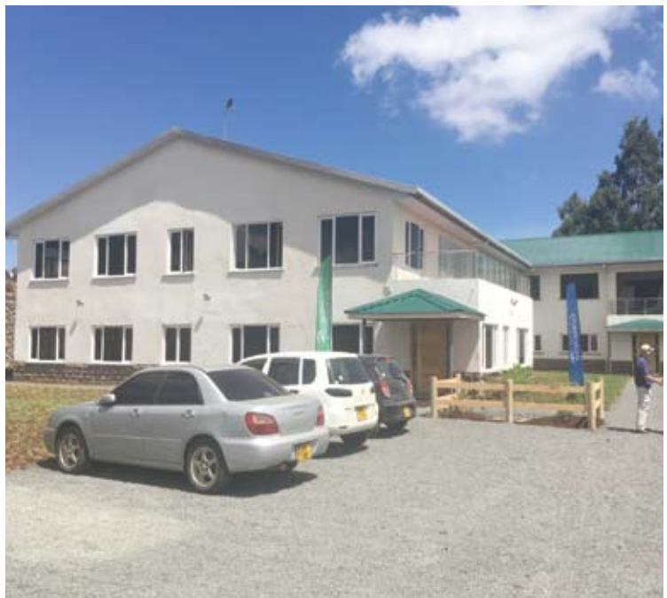
The new CropNuts home located in Limuru town in Kiambu County that has a spacious area with growing facilities to offer a wider range of analytical and technical services
