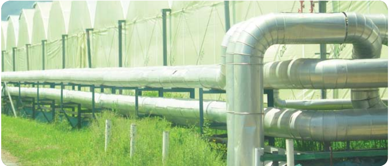
Greenhouses at Oserian. The farm runs the world's largest geothermal greenhouse heating project to reduce carbon emissions and control climate.
